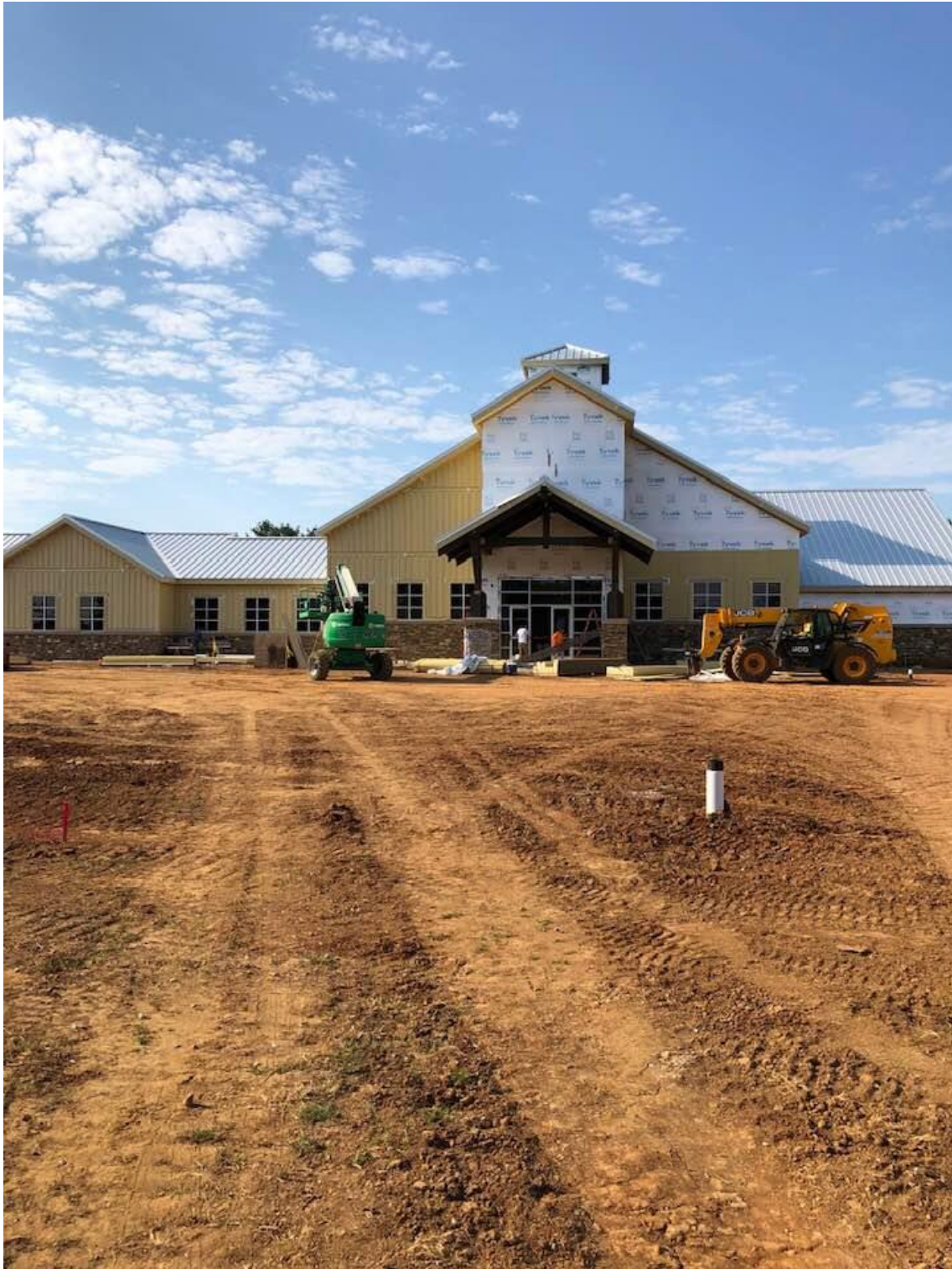
Work continues on the National Museum at the SCV Headquarters at Elm Springs in Tennessee
